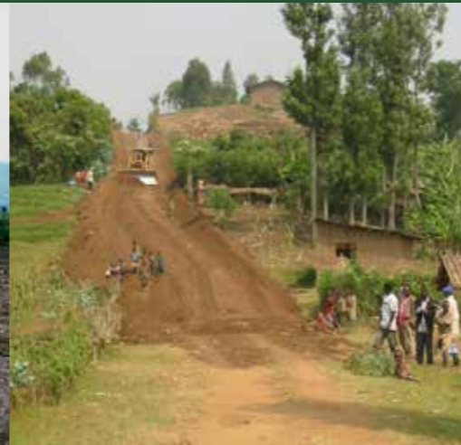
Building the 4 km road
