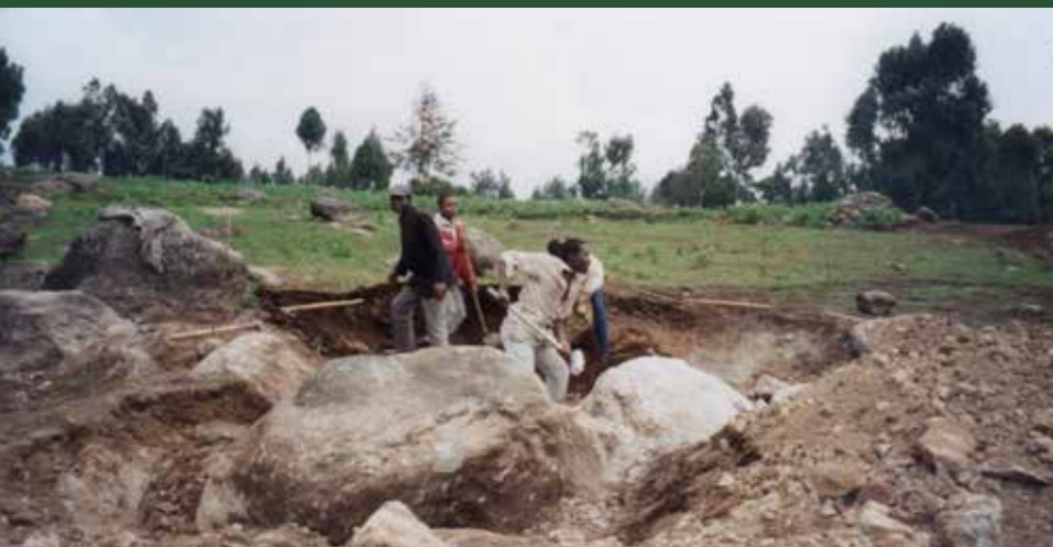
Preparing the site
