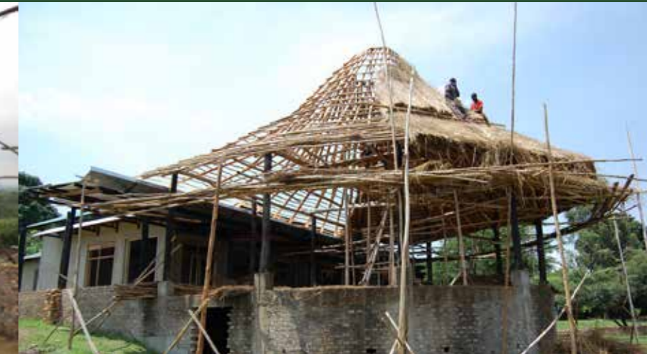
Building of the sombrero
