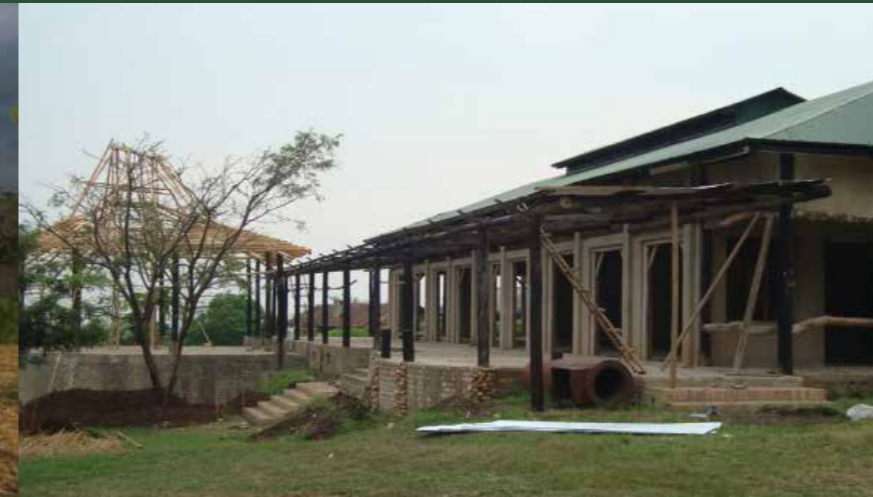
Main building remodelling
