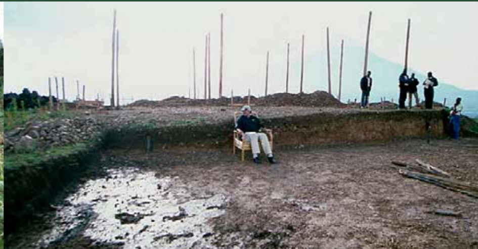
Praveen overseeing foundation work
