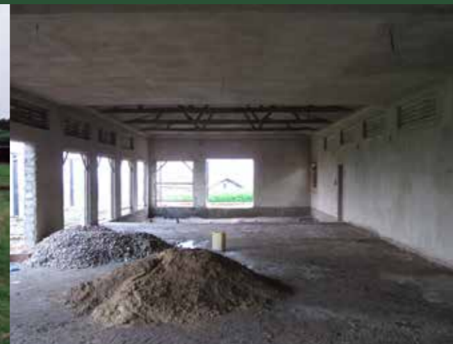
Renovating the old coffee shed
