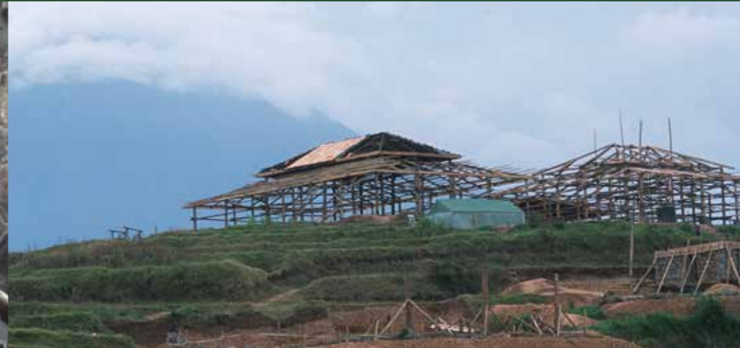
Building the public areas
