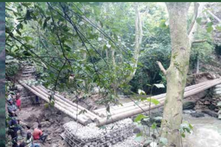
Building bridge across river
