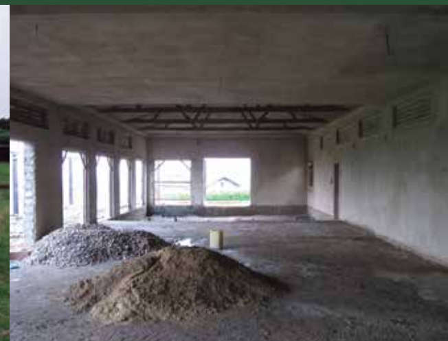
Renovating the old coffee shed
