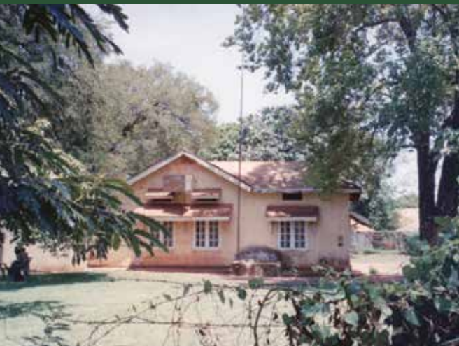
Post Master's house in Masindi
