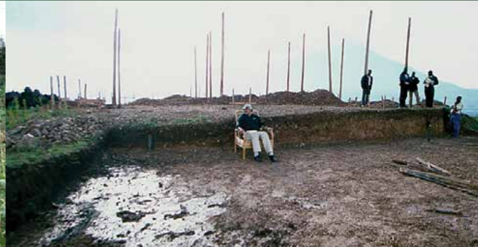
Praveen overseeing foundation work
