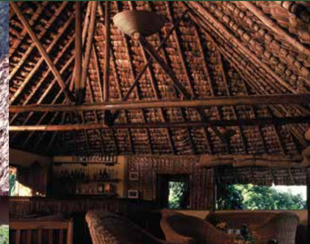
Roof of living room
