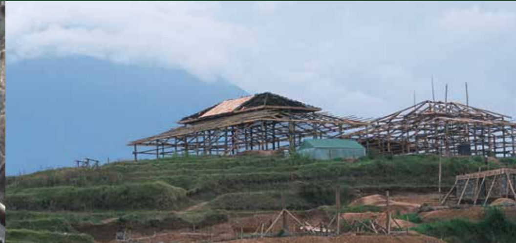
Building the public areas
