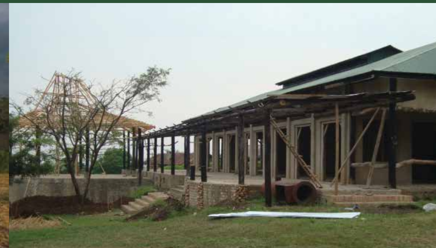
Main building remodelling
