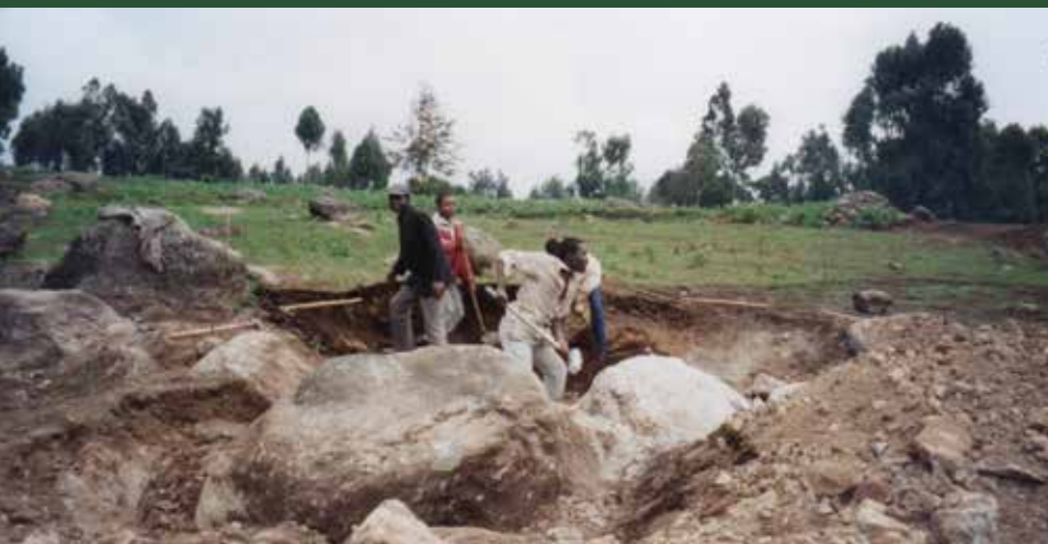
Preparing the site
