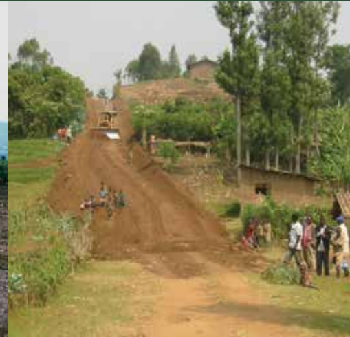
Building the 4 km road
